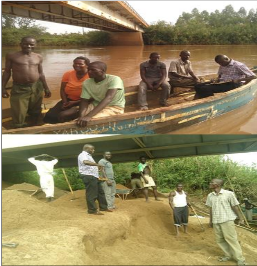
Plate 3.4: Sand harvesting at Rwambwa bridge
